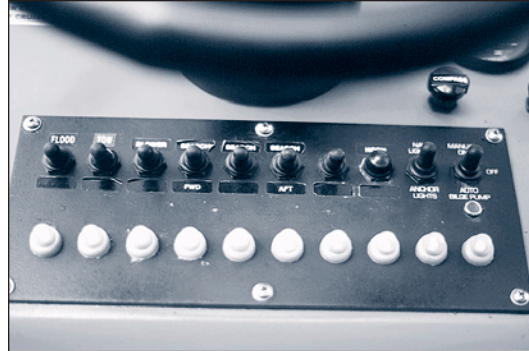
Each crew member should be familiar with controls
